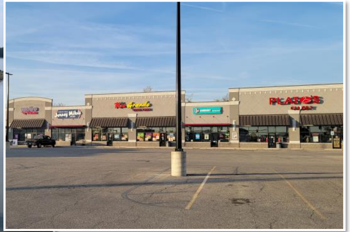
4315 Milan Road - Perkins Township
