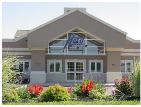
Hoty Enterprises office - Perkins Twp.
